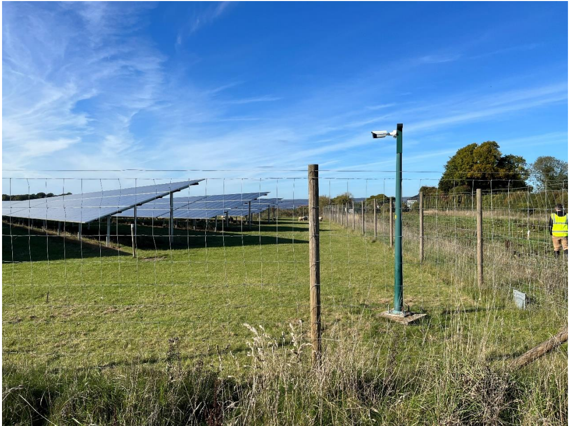
Plate 2-7: Stock Proof Fencing and CCTV pole
