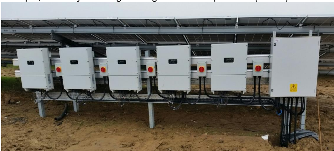
Plate 2-3: Typical string inverters installed under PV modules
