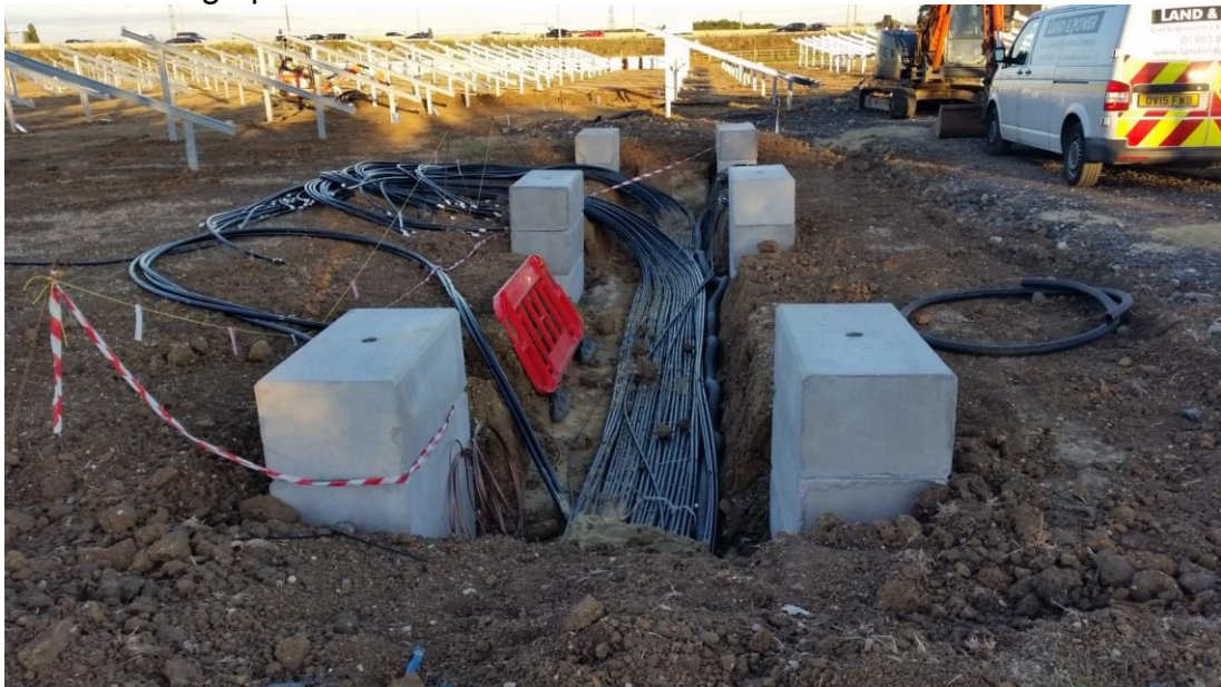
Plate 2-6: Example underground cable installation
