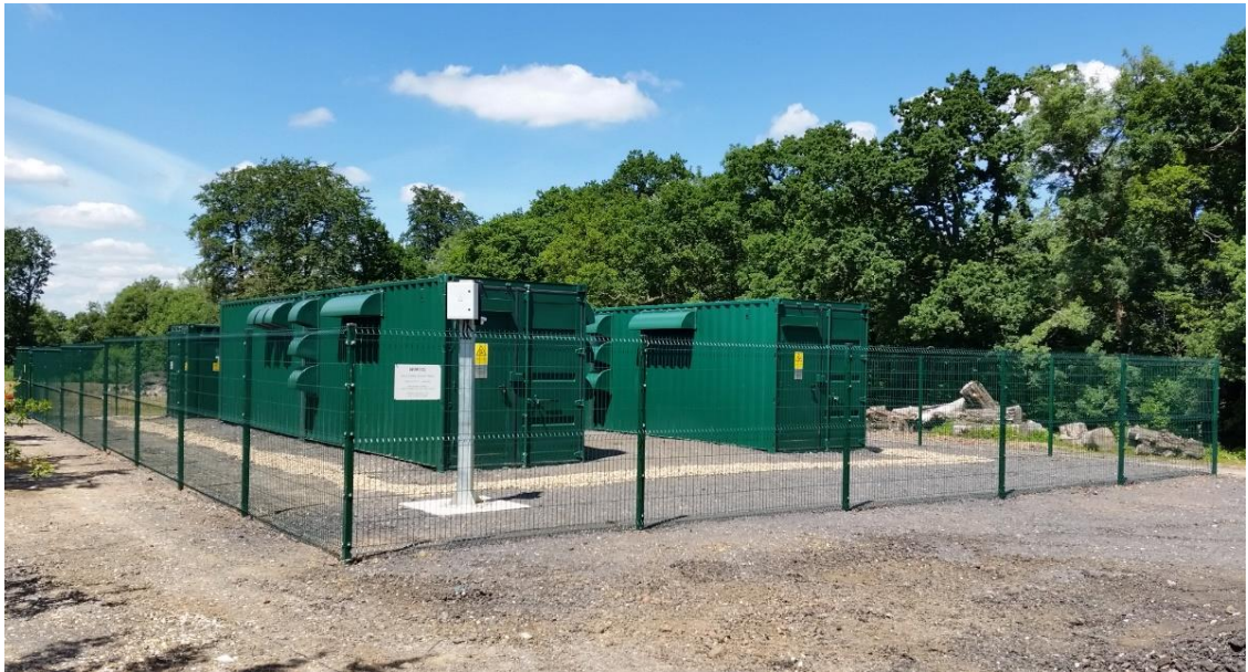
Plate 2-4: Typical central inverters
