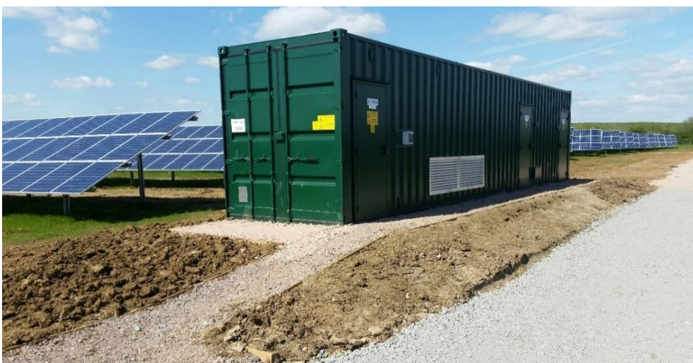
Plate 2-5: Example MV station
