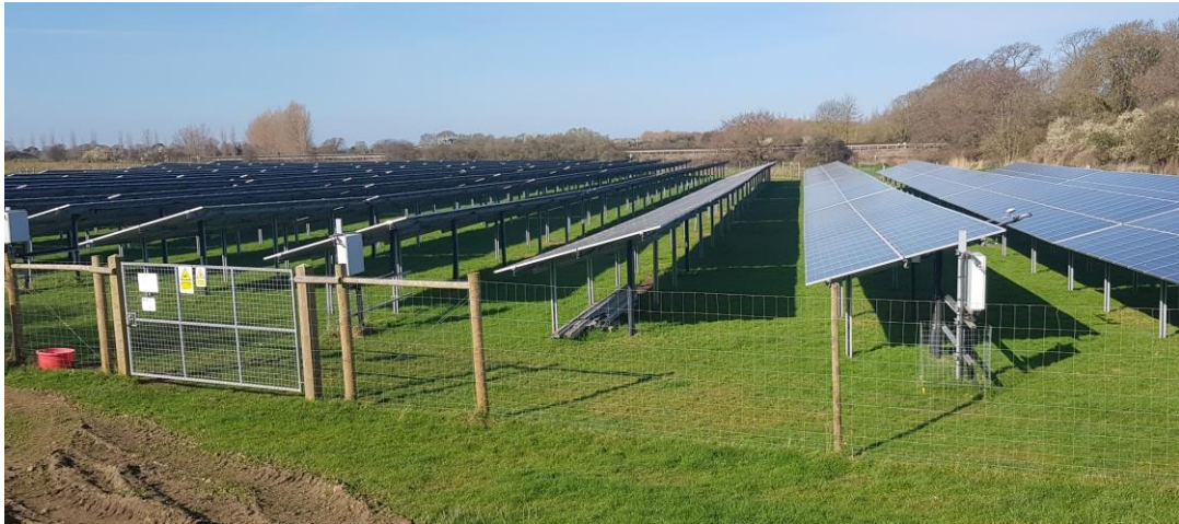
Plate 2-1: Fixed tilt modules, finished array
