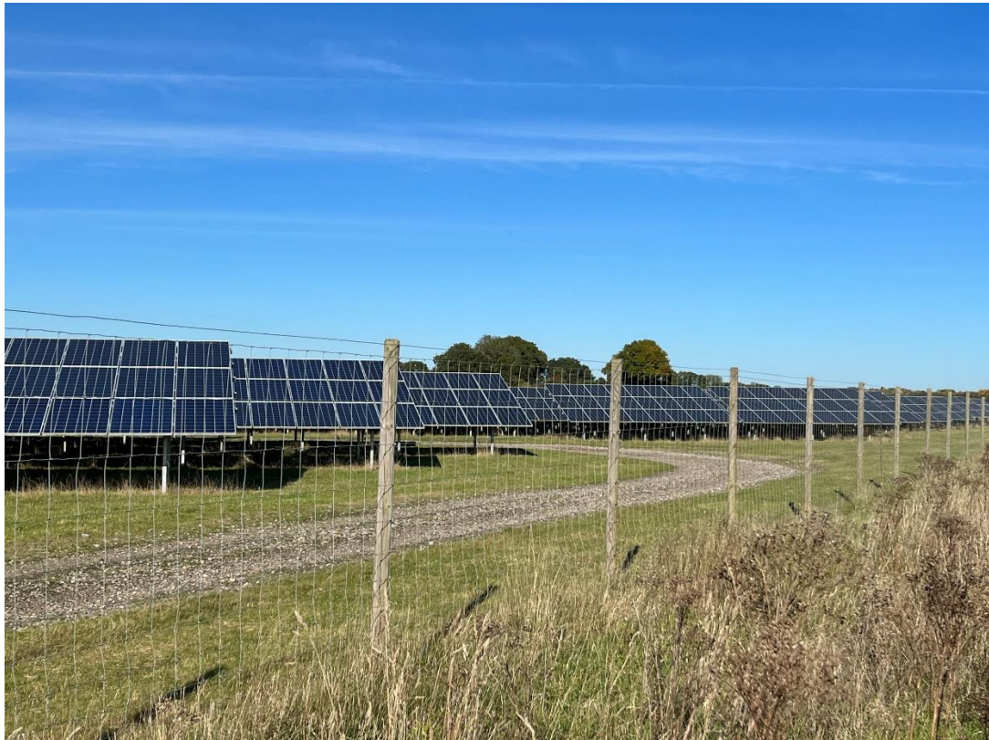
Plate 2-8: Typical crushed stone access track laid on hardcore and geotextile
