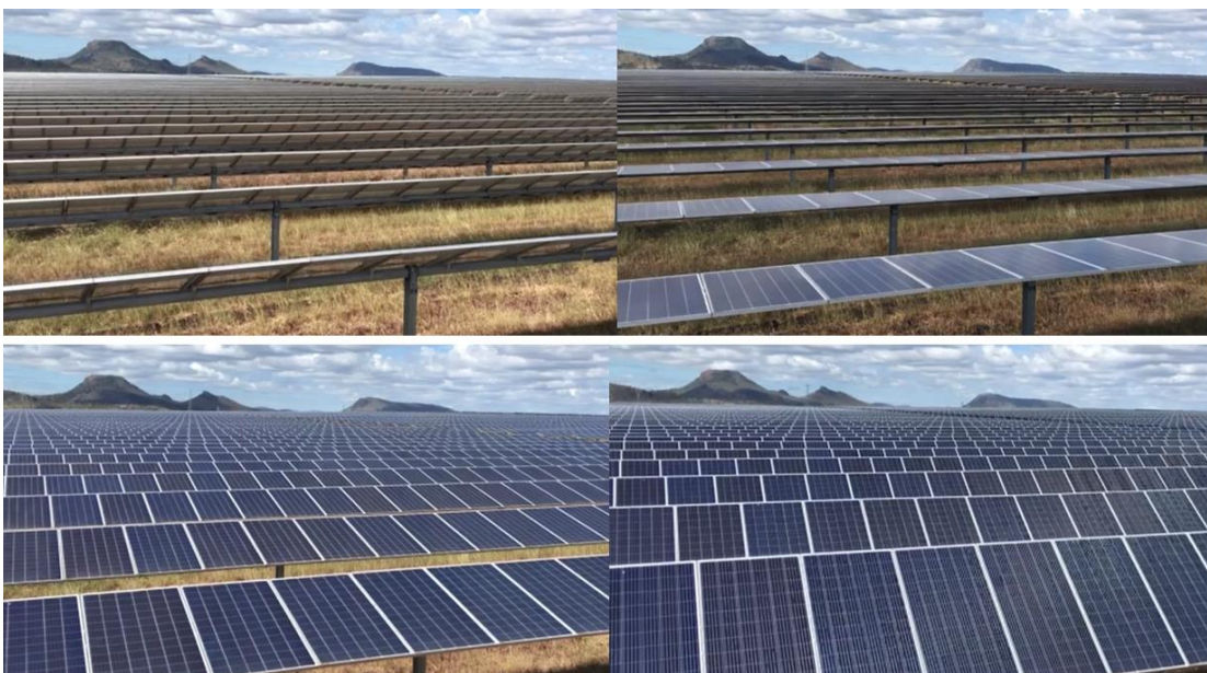
Plate 2-2: Single axis tracker system, finished array
